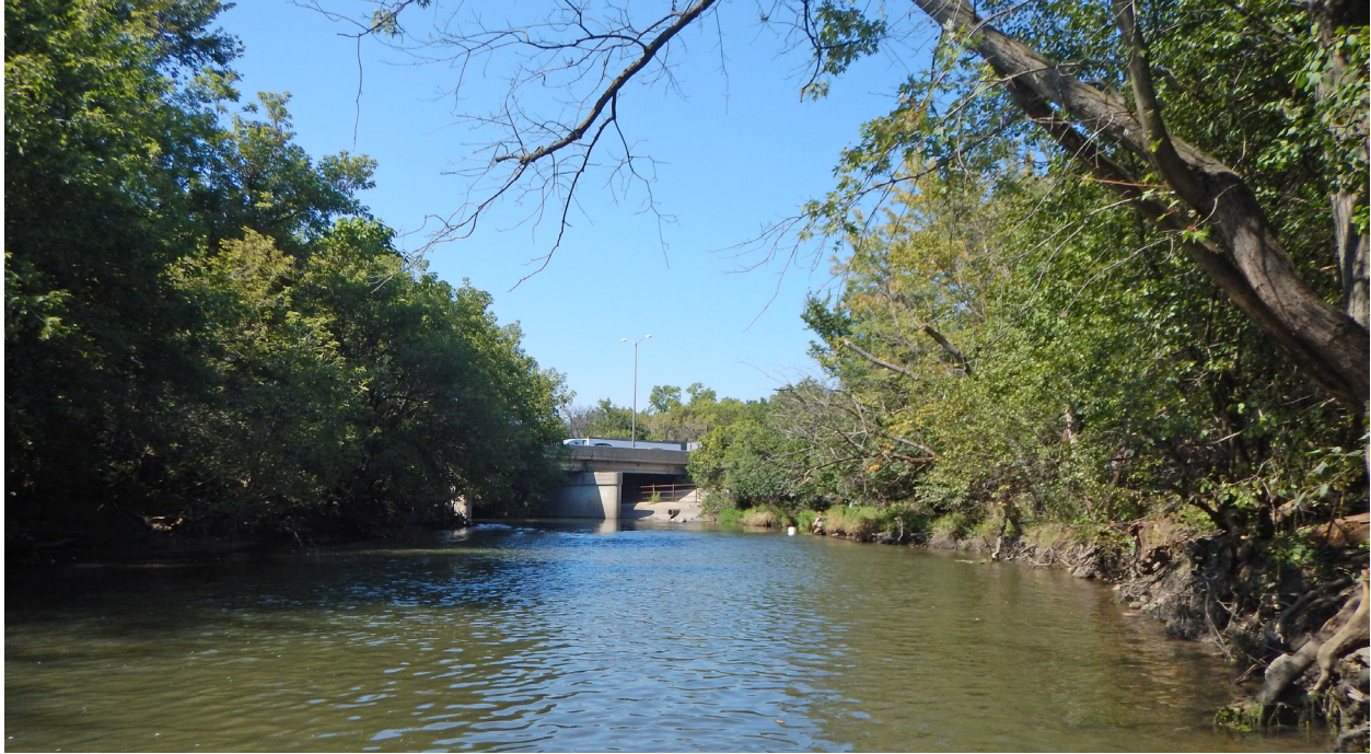
PLATE 4. Salt Creek at I-294 (Cook County, IL) taken from near bottom of reach looking upstream at I-294 bridge. Photo by E. Bilger.
