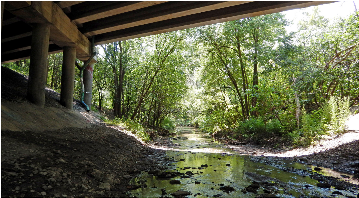
PLATE 6. Site photo of Flag Creek at Spring Rock Creek Park (Cook County, IL) with 47 th Street Bridge. Photo by E. Bilger.
