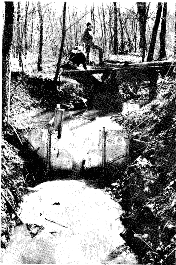
Figure 9. Outflow weir at Heron Pond
