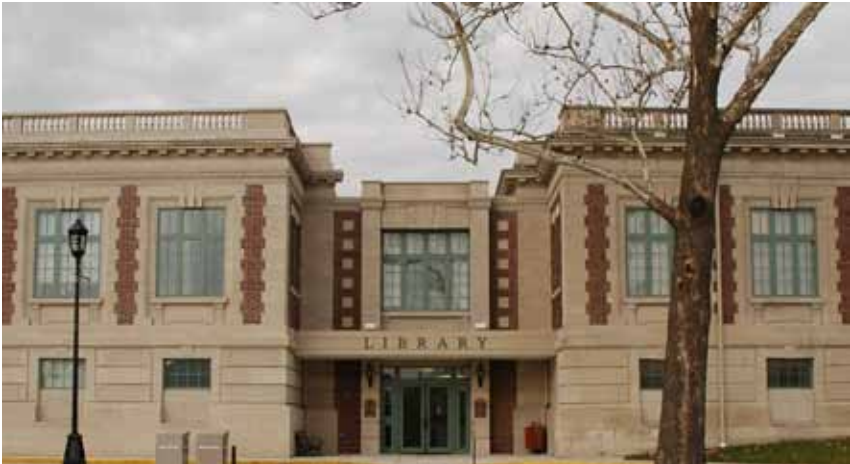
Figure 4. The brickwork of the new wing of the expanded LaSalle Public Library closely matches the building's original brickwork, but any difference is made less noticeable by separating the two areas of brickwork by the new, accessible entrance. The original building is on the right. Photograph courtesy of apaceDesign, architects and engineers, Peoria.
