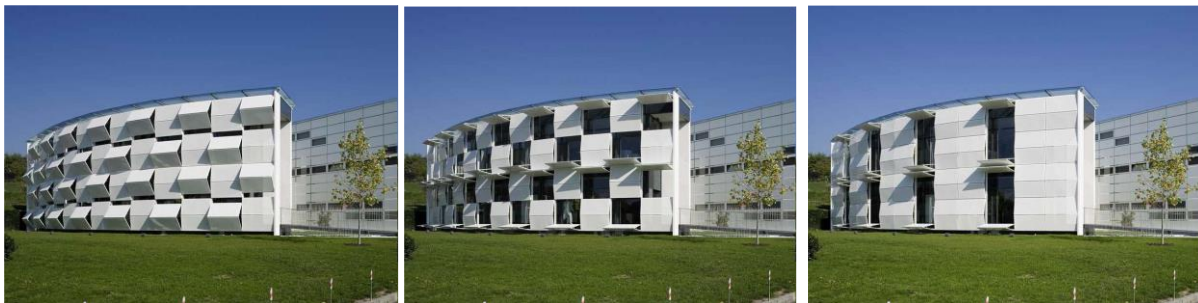
Figure 2.4: Dynamic façade; Kiefer Technic showroom Bad Gleichenberg Giselbrecht (pictures by Paul Ott).
