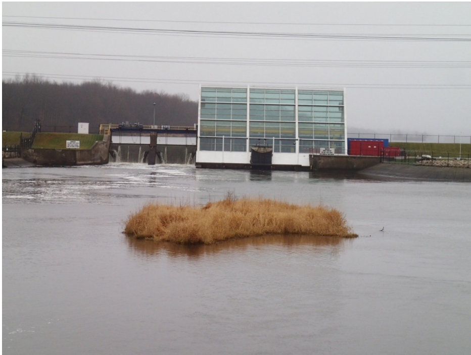
Figure 2.8: Structures at the Morrow Dam
