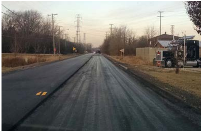
Figure 25. Typical tack coat installation; note zebra pattern.
