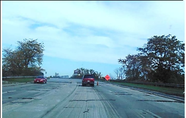
Figure 12. Segment 3 (159th Street to I-57) cold-milled pavement.
