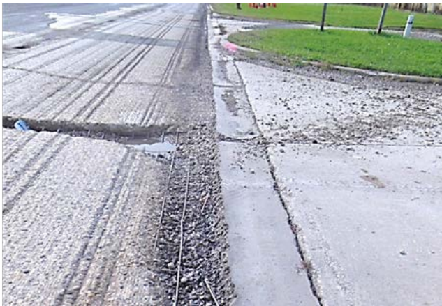
Figure 11. Segment 3 (159th Street to I-57) cold-milled pavement.
