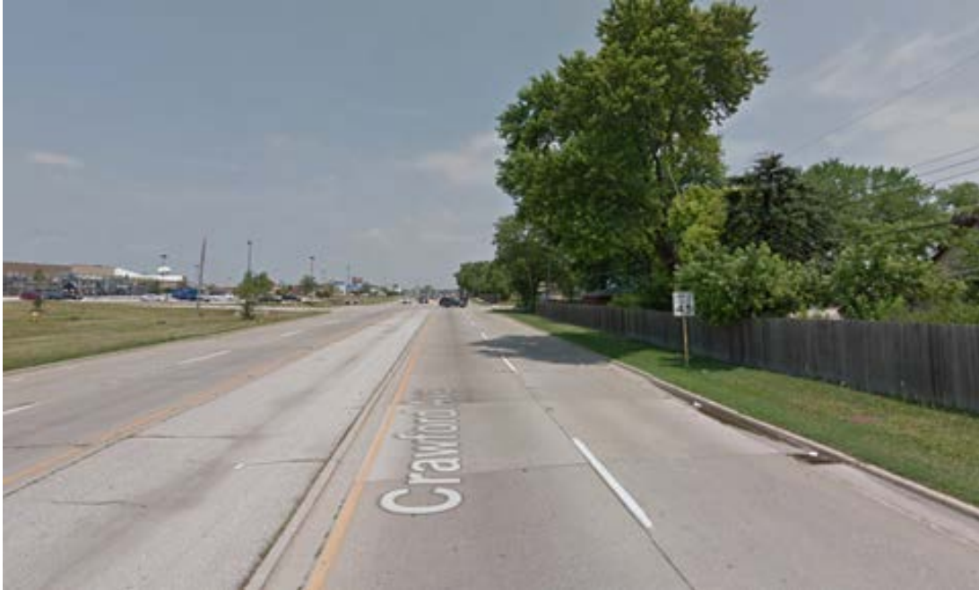
Figure 3. Segment 2 of Crawford Avenue/ Pulaski Road looking north to 169th Street (image: Google).
