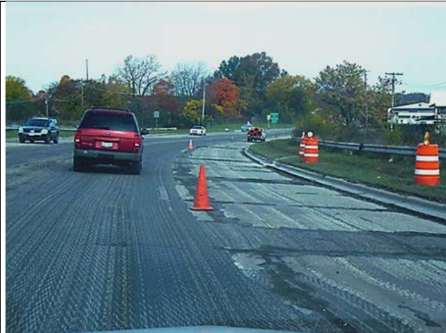
Figure 9. Segment 3 (159th Street to I-57) cold-milled pavement.
