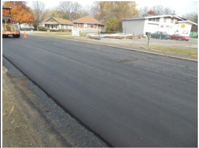
Figure 24. Level course installed 1 ft narrower than cold-milling operation.
