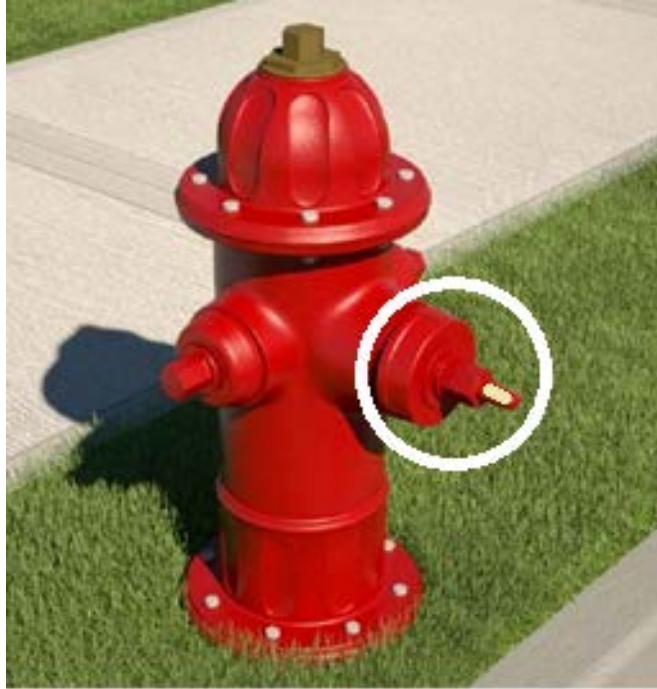
Figure 2.6 Fire hydrant equipped with the acoustic monitor node.
