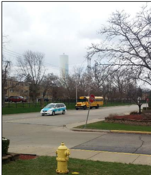
Figure 2.2 Linneman Road standpipe, Waycinden, Illinois.
