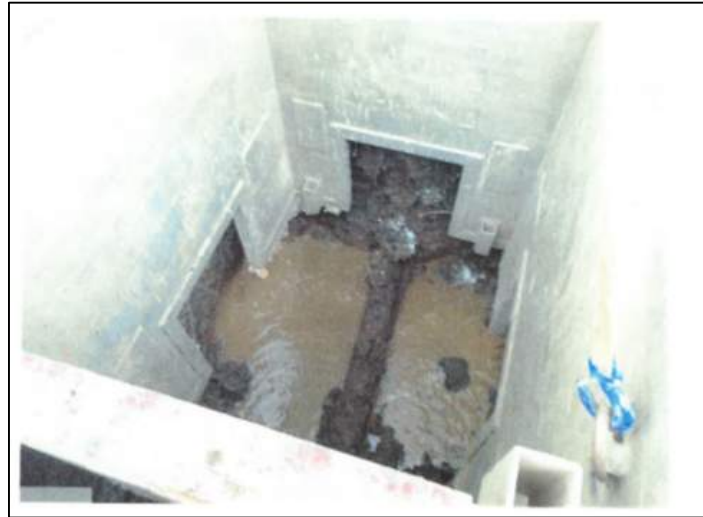
Figure 3.13 Leak repair at 1181 Stark Place.
