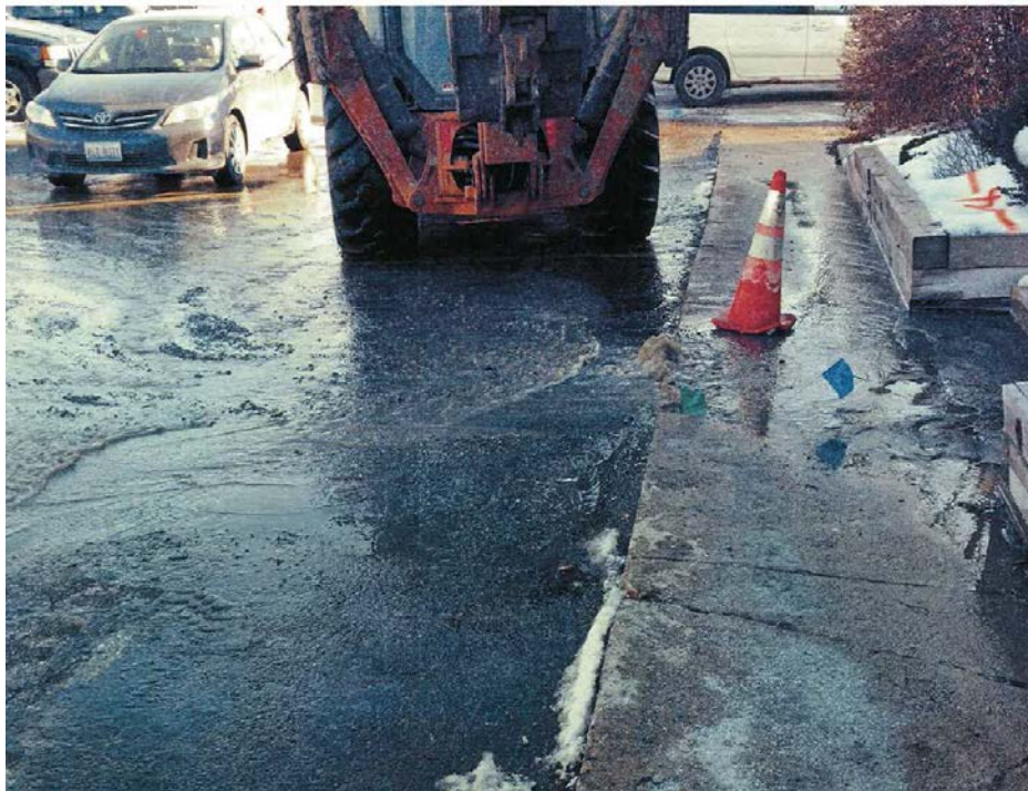
Figure 3.19 Leak surfacing 724 Algonquin Road.
