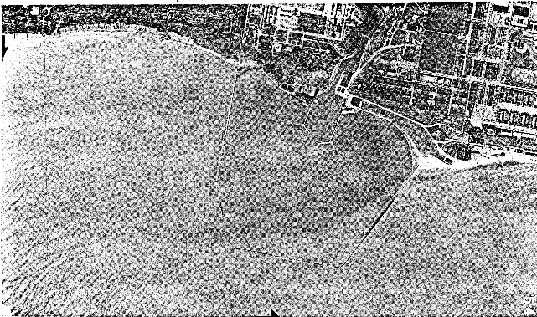
Fig. 15 - Great Lakes Naval Training Center harbor in April, 1958 showing wave fronts from the northeast. At the south end of the north fillet, waves break over the north jetty depositing sediment within the harbor. Natural flow extends along the inside of the north and east jetties toward the mouth of the harbor. Small wind-induced waves are present over the shallowest part of the harbor fill just inside the east jetty. Reflected wave patterns can be seen in the north fillet area as well as off the distal end of the east jetty. Refracted waves curl around the south side of the harbor.
