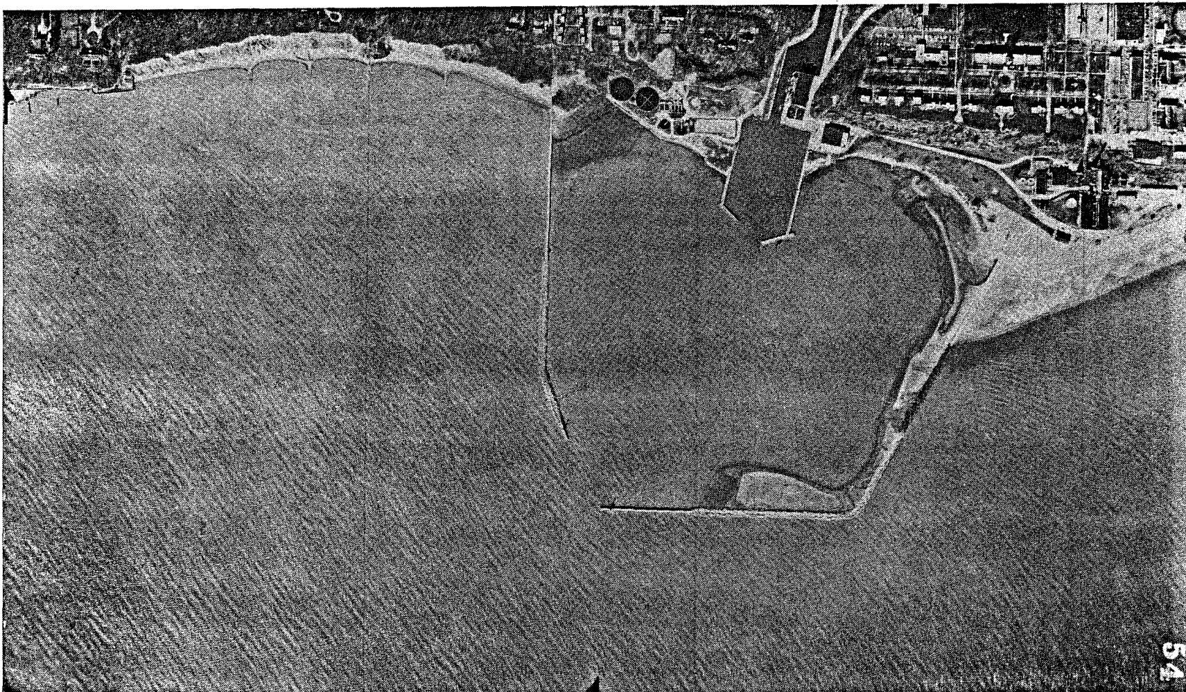
Fig. 14 - Great Lakes Naval Training Center harbor in April 1964 showing emergent north fillet and harbor filling at abnormal low water levels. Waves from the southeast show wave reflection patterns adjacent to the landward end of the south jetty as well as at the distal ends of the south, and east jetties. Refracted wave fronts are seen within the harbor and adjacent to the north fillet.
