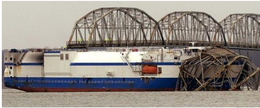
Figure 90. A cargo ship collision in 2012, causing Eggner Ferry Bridge, KY, collapse.
