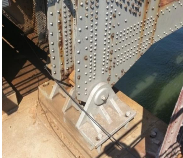
(c) The boundary condition of the bridge.
