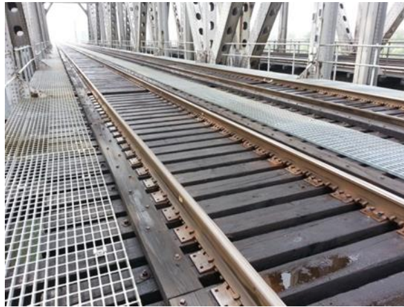
(a) Track system, rail, and fastening.
