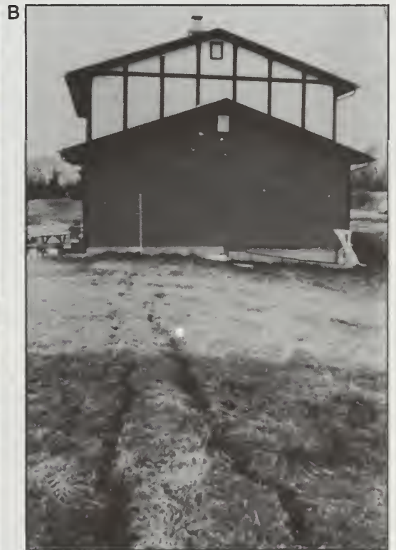
Figure 9 Block diagram and photos of a typical sag subsidence event. A. Road in compression zone. Asphalt has buckled. B. Wood frame house in tension zone. Foundation has pulled apart and dropped away from the superstructure in one corner. C. Brick house in tension zone. Walls, ceilings, and floors have cracked.
