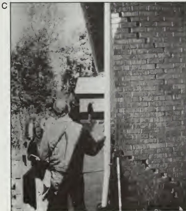
Figure 9 Block diagram and photos of a typical sag subsidence event. A. Road in compression zone. Asphalt has buckled. B. Wood frame house in tension zone. Foundation has pulled apart and dropped away from the superstructure in one corner. C. Brick house in tension zone. Walls, ceilings, and floors have cracked.
