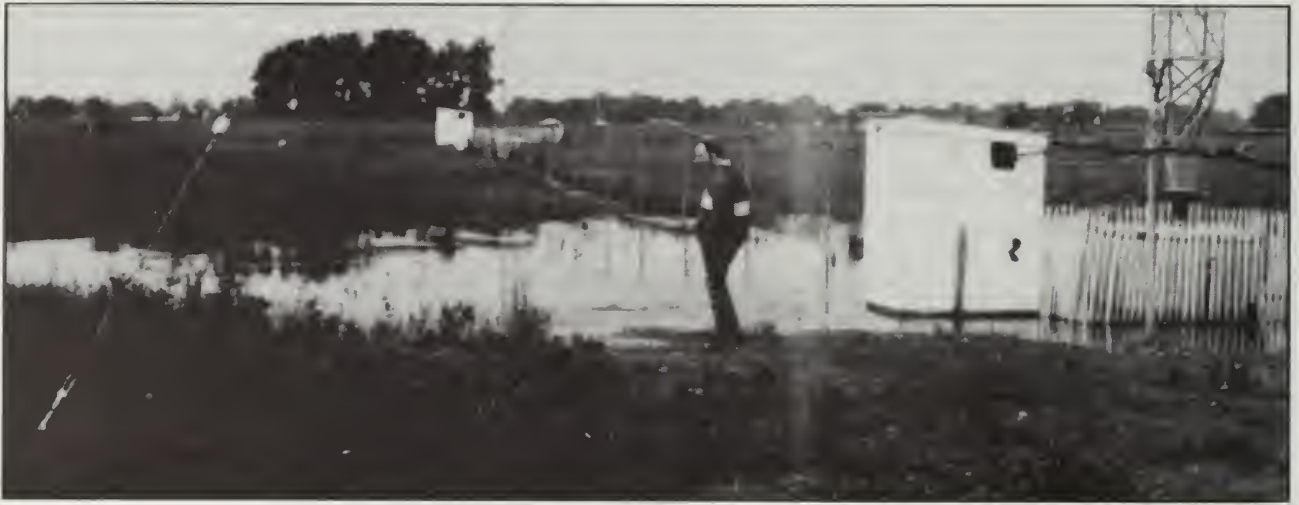
Figure 12 Ponding created by sag subsidence.
