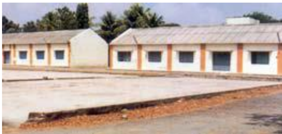
Figure 2.14 Brick-build Godowns (Joshi 2002)
