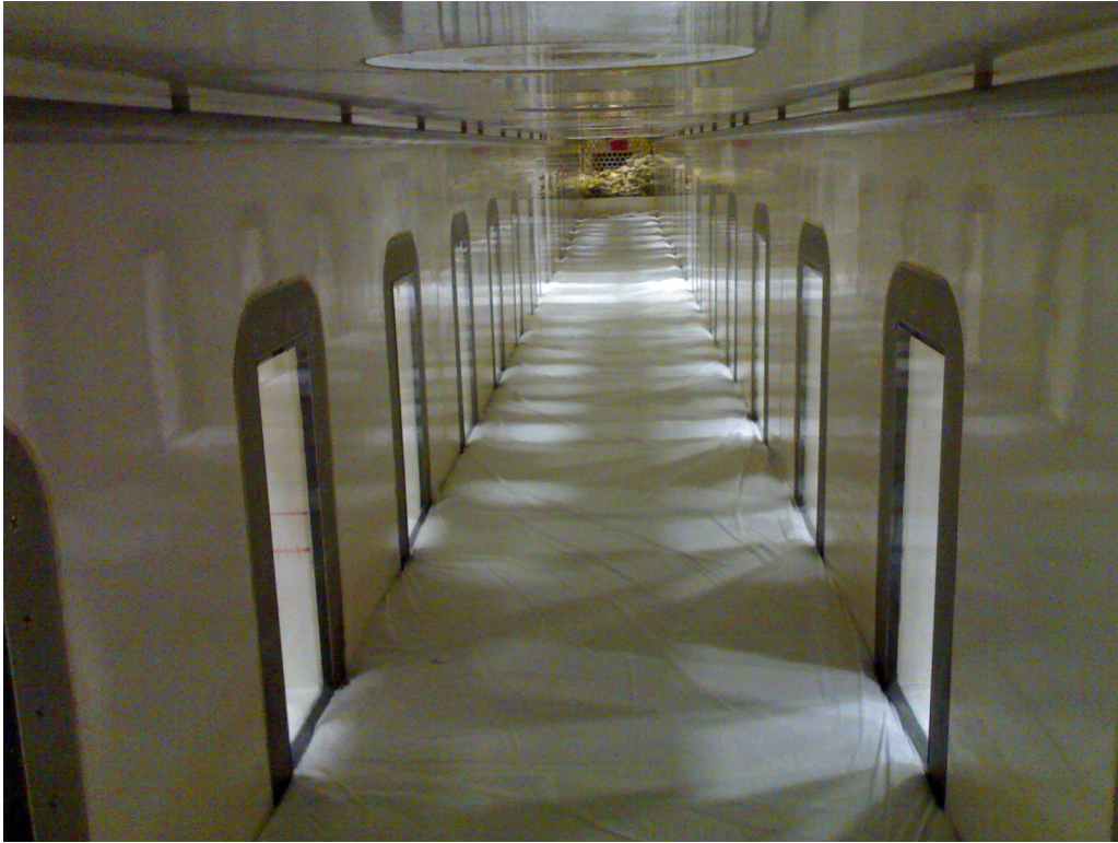
Figure 39. Picture of the inside of LOWST after sand extraction, with the fine-mesh geotextile in place.
