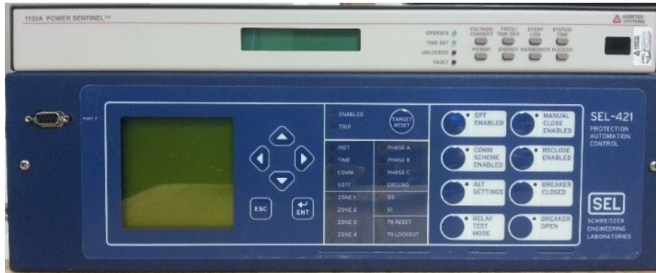
Figure 2.2: Two phasor measurement units from the TCIPG testbed at University of Illinois at Urbana-Champaign.
