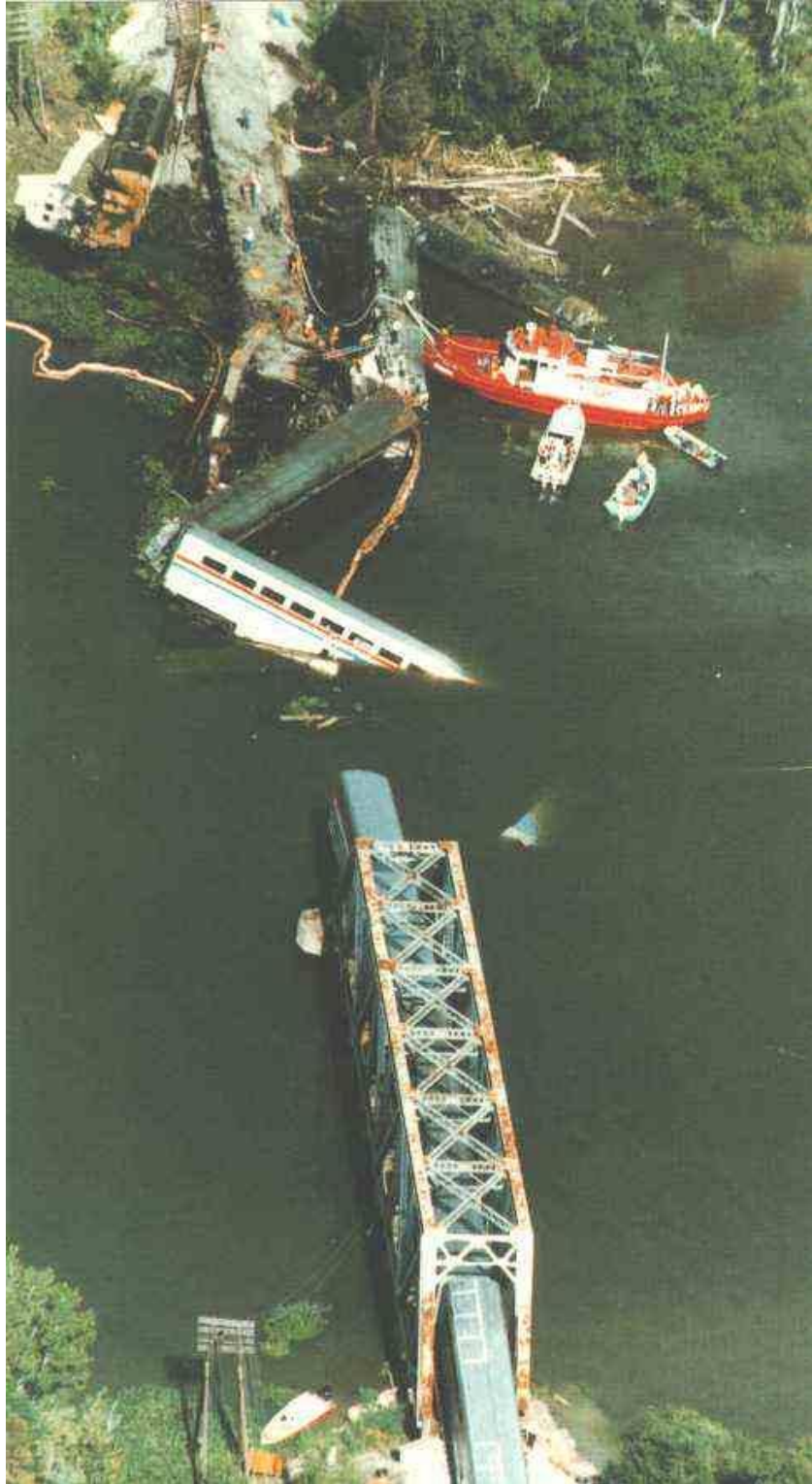
Figure 2.9. Alabama bridge accident, 1993 (Gendisasters.com, 2014)
