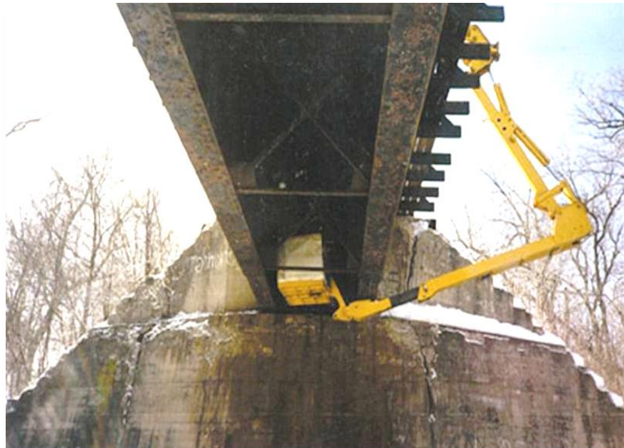
Figure 2.5 Railroad bridge inspection conducted from the railroad track (Sweeney and Unsworth, 2008)
