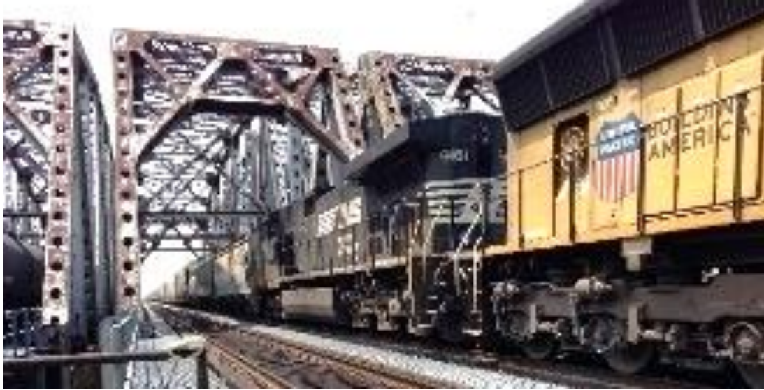
Figure 2.10. Railroad bridge under revenue service traffic.
