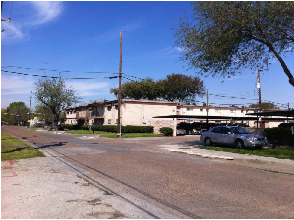
Photo 6.4: Granada Terrace Apartments
