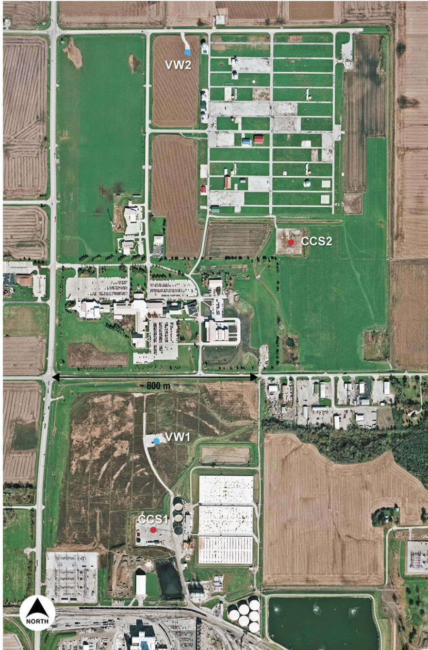
Fig. 1.1. Aerial site photo of the IBDP. CO 2 is compressed into the supercritical state, transported 1 mile along a pipeline, and injected into the CCS#1 well at a depth of ~7,000 ft. (2,134 m) into the Lower Mt. Simon Sandstone.
