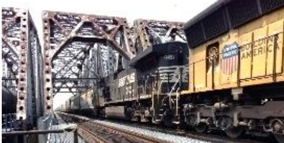
Figure 2.10. Railroad bridge under revenue service traffic.
