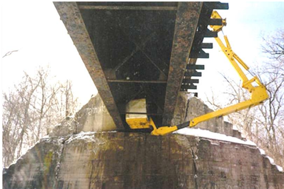
Figure 2.5 Railroad bridge inspection conducted from the railroad track (Sweeney and Unsworth, 2008)
