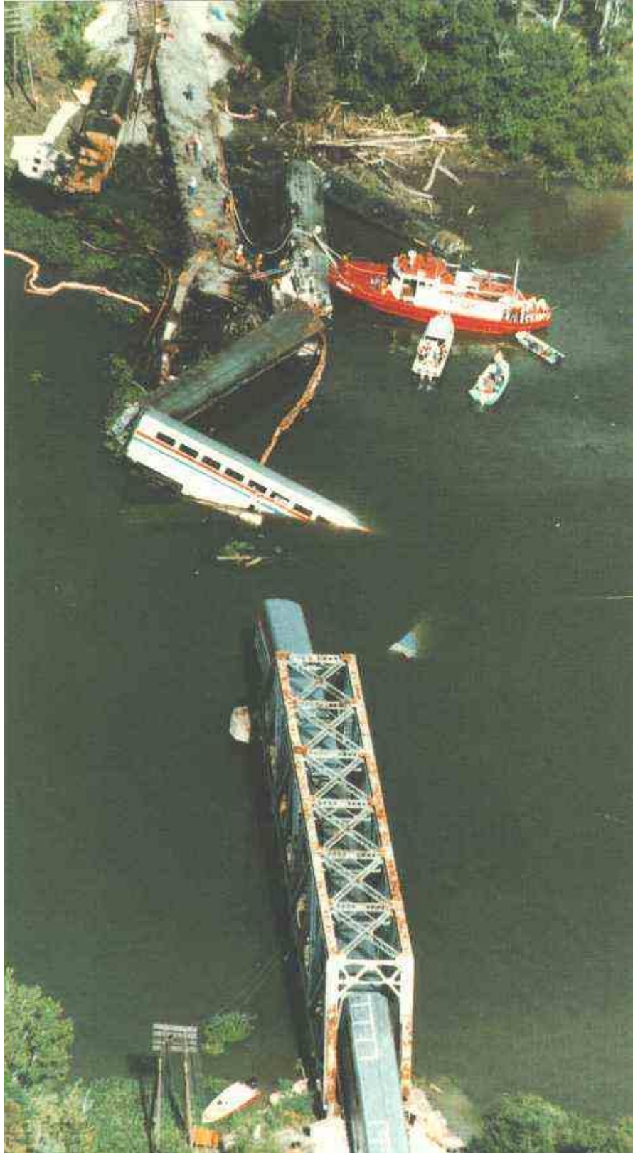
Figure 2.9. Alabama bridge accident, 1993 (Gendisasters.com, 2014)
