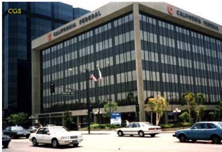
Figure 7.2 A six-story building in Burbank, California
