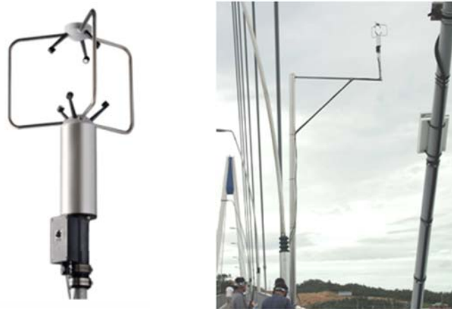
Figure 0.91. RM Young 8100 ultrasonic 3D anemometer (left) and installation on girder (right).
