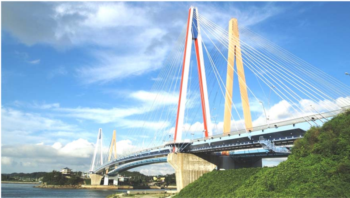
Figure 0.81. The Jindo Bridges.
