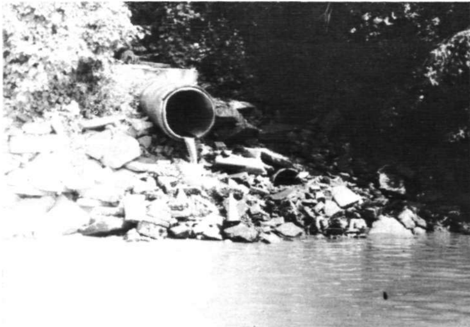
Figure 5. Washington Street outfall
