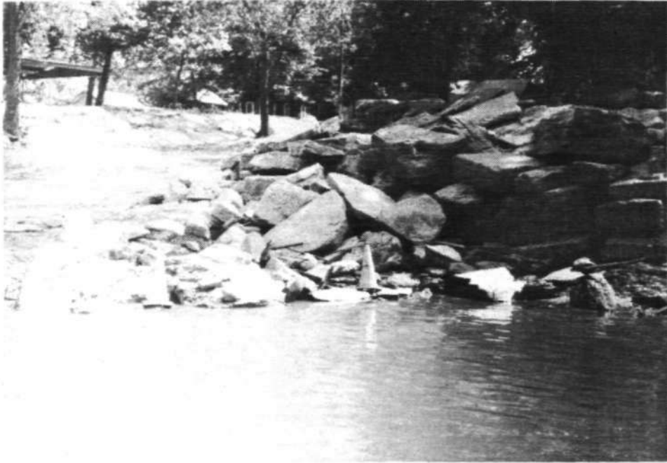
Figure 4. Market Street outfall area
