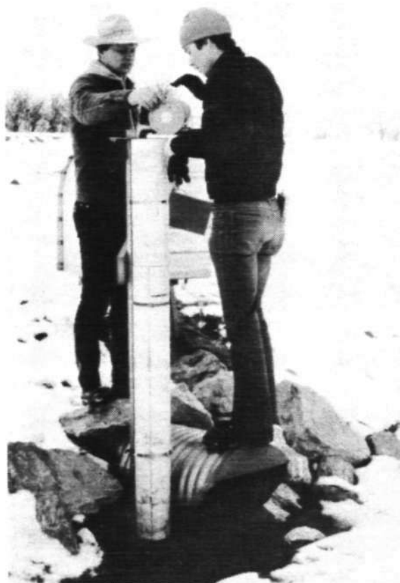
Figure 4. Installation at Field Site 2
