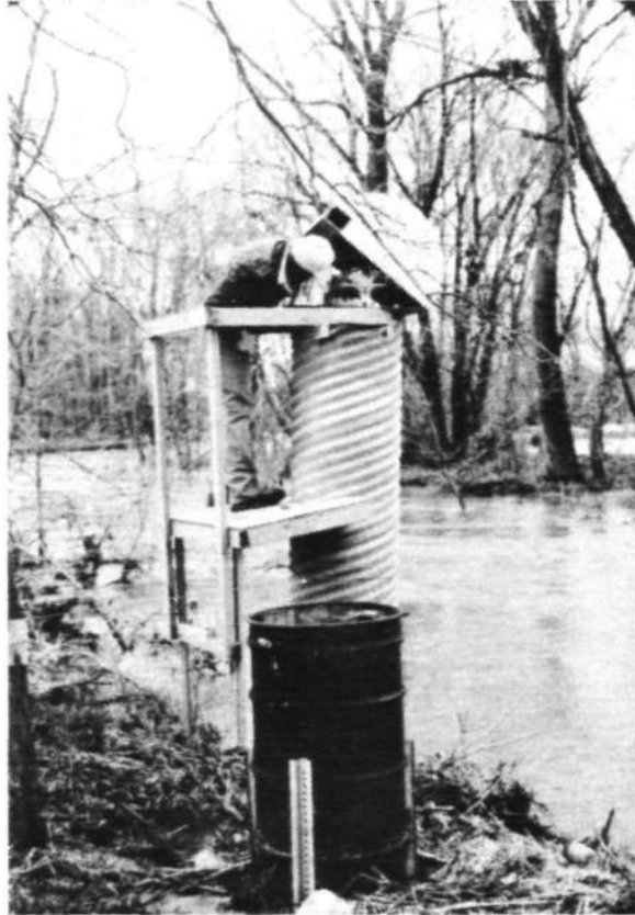
Figure 5. Typical streamgaging station installation with stage recorder on top of the stilling well and automated sampler in the foreground (Note that the creek is at bankfull flow)
