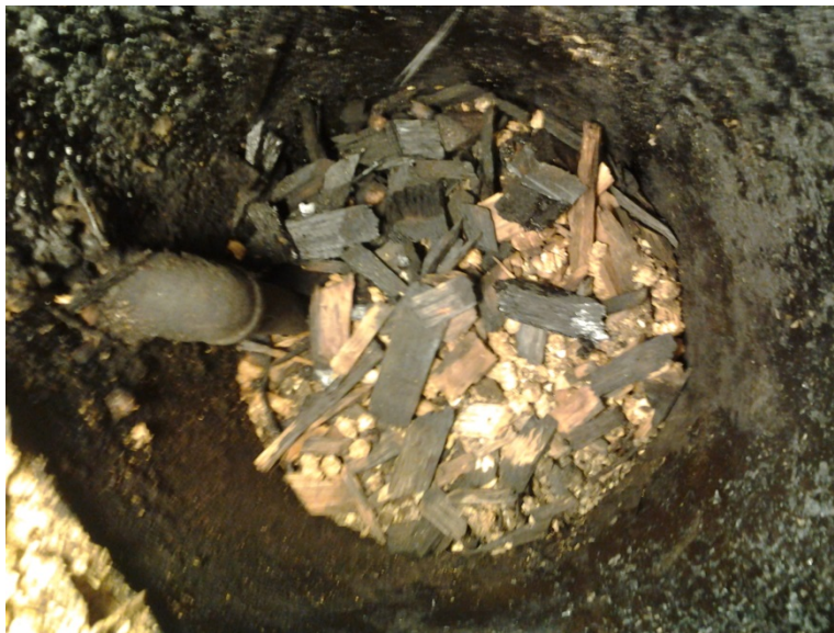
Figure 15. Switchgrass pellets were seen segregated from wood chips, approximately 12 inches from the top of the reactor.
