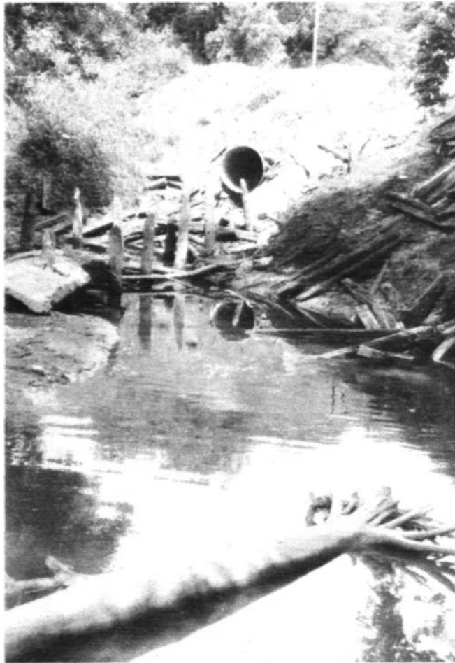
Figure 15. Close-up of Fayette Street outfall pipe
