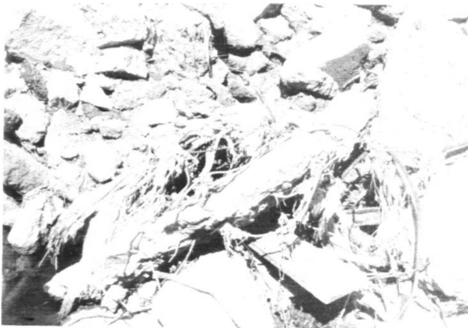
Figure 14. Close-up of debris collection in Court Street outfall channel
