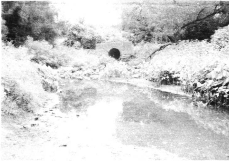
Figure 2. State Street outfall
