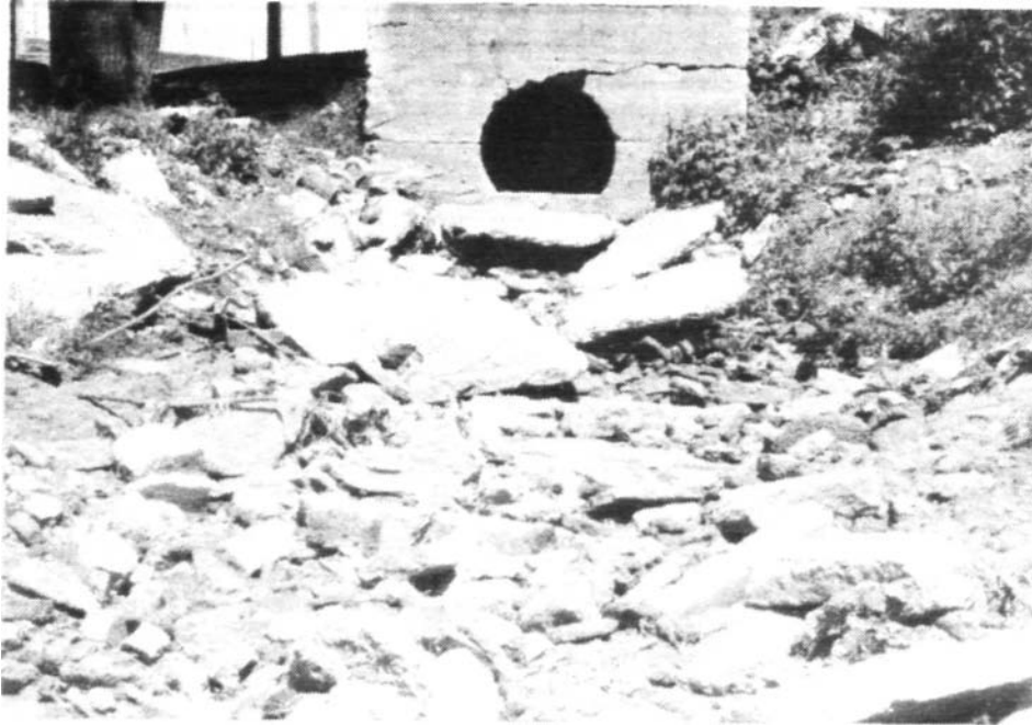
Figure 13. Close-up of Court Street outfall channel
