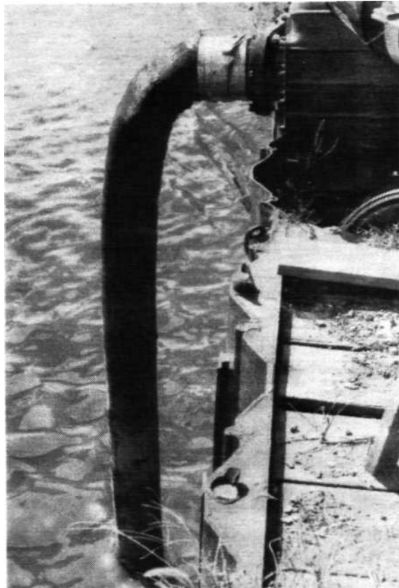
Figure 3. Pump installation at Cedar Street, showing suction line
