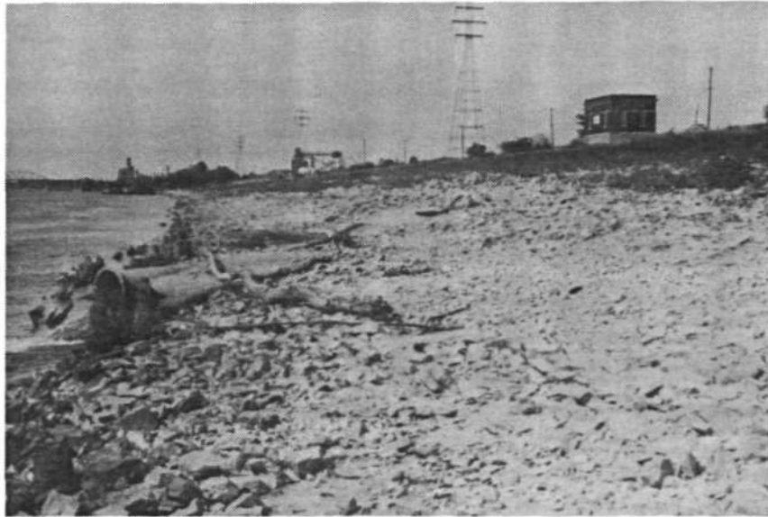
Figure 10. Outlet of stockyard gravity line
