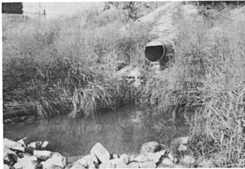
Figure 11. Outlet of Hi-line
