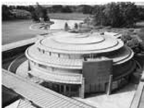
Aerial view over Francis Crick Auditorium and the Genome campus
