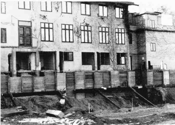
Renovation of Blackford Hall
