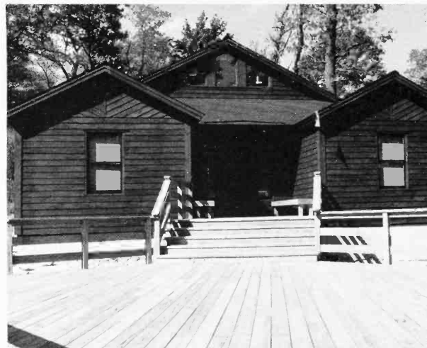
One of five new cabins under construction
