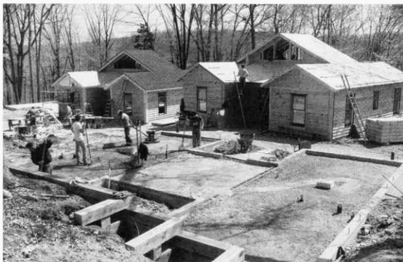
Cabin Complex under construction
