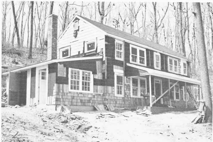
Urey Cottage under renovation
