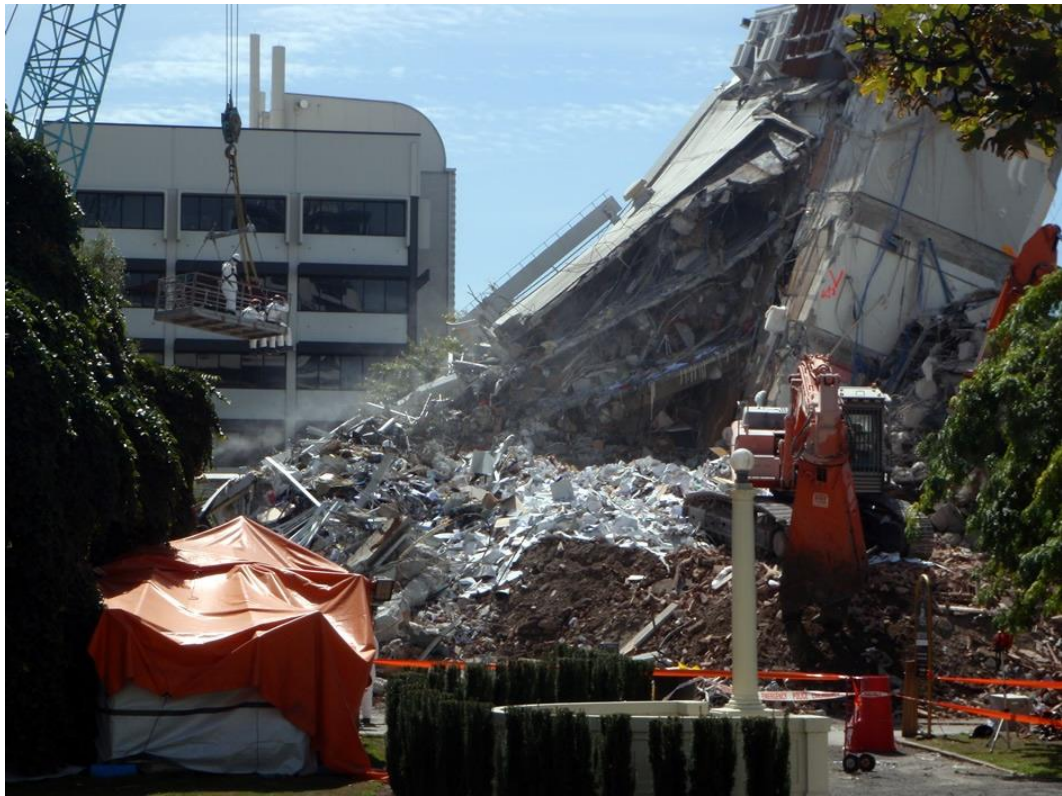
Figure 1.1: PGC building collapsed (Ministry for Culture and Heritage, 2011).
