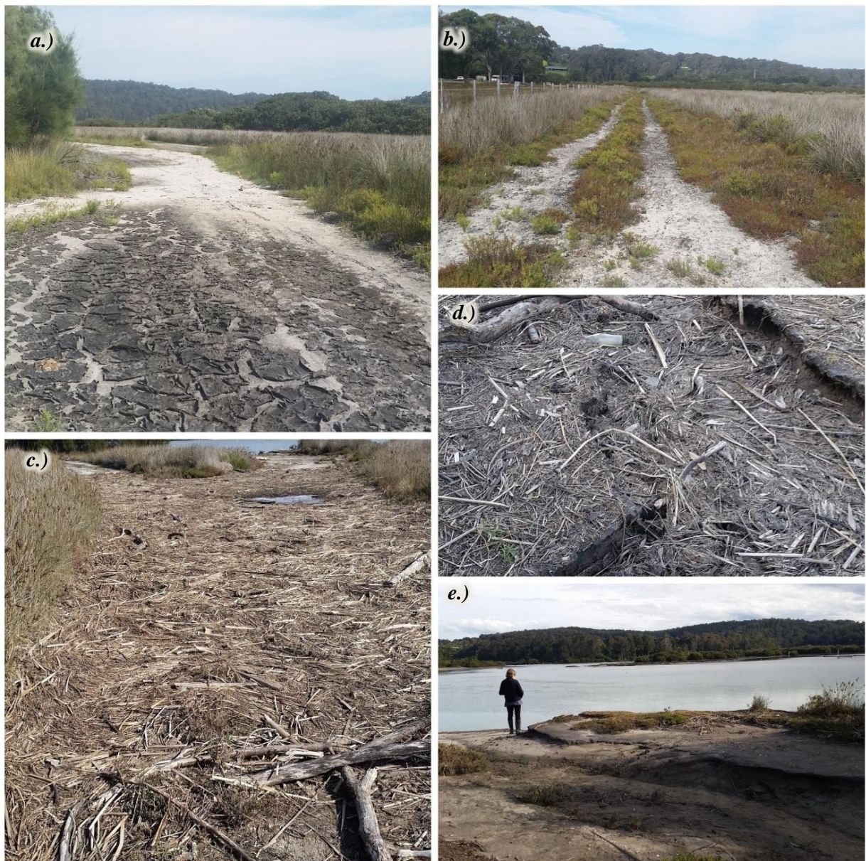
Figure 8: Vehicle damage at Bermagui
