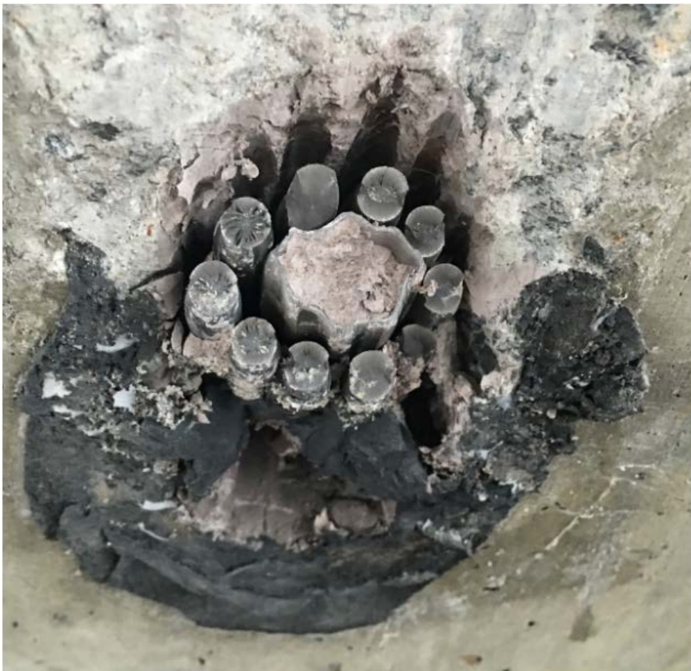
Figure 7: Cross sectional view of Cable bolt Unbulbed, Plain MW10, 15 t pretensioned and debonded. Note the extent of wire failure in tension of Cone and Cup. The failure load of 68.2 t is almost equal the cable axial load capacity of 70 t. The shear load displacement at failure was 68.2 mm.
