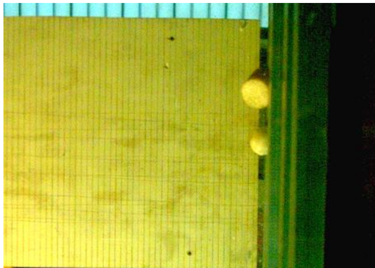
Figure G.2: Pictures of the impact on corrugated steel sheet
