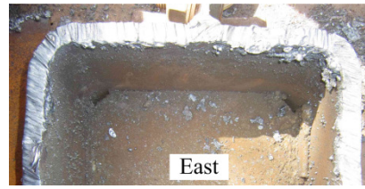
(b) Well fabricated welding on the east side.
