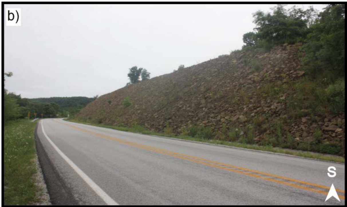
Fig. 5 Riprap with steep angle of repose, part of the most recent mitigation effort to a historically problematic failure zone along Arkansas Highway 7, looking north toward Jasper (a) and looking south uphill (b) with the summit of Round Mountain immediately west
