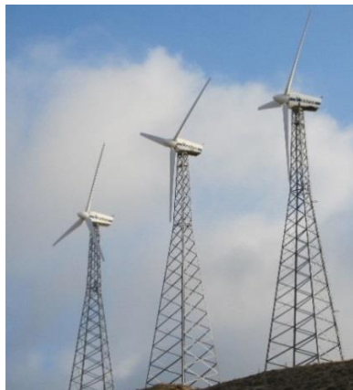
Figure 1-7. Lattice tower (Big Stone Renewables Services)
