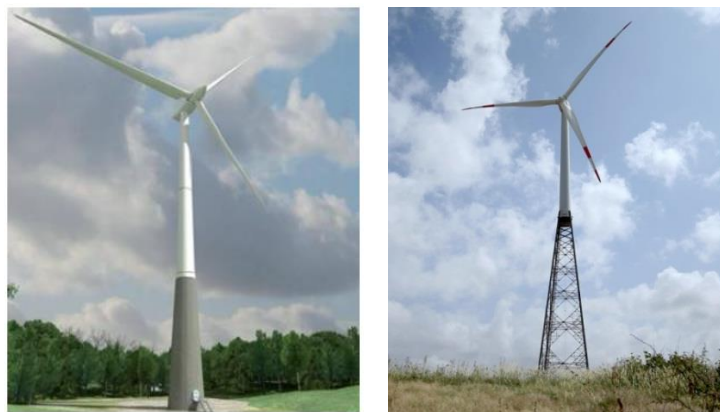
Figure 1-10. Hybrid tower (Ozturk, 2016)
