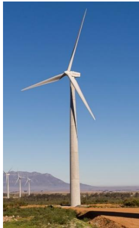
Figure 1-8. Concrete tower (Florez, 2015)
