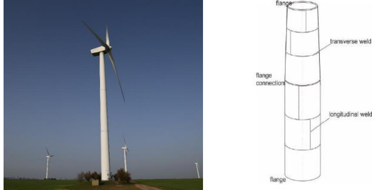
Figure 1-9. Tubular tower (Tackle TW 1.5S)
