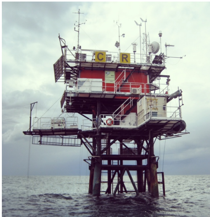
Figure 1 – The ISMAR oceanographic tower, 15 km offshore the coast of the Venice lagoon, in the northern Adriatic Sea, East of Italy (see Figure 2). The upper structure has now been replaced by a new, two metre higher, one.
