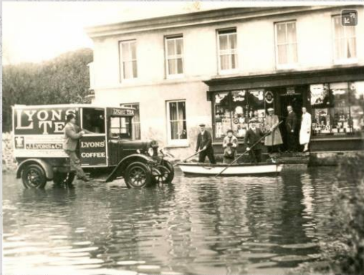
Flooding on Brooks Corner, this was commonly paired with flooding on Harbour Road
