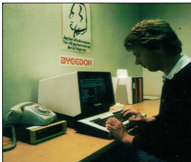
Figure 4.19 Byggdok online access by means of 1,200 bps modem in the 1980s.
