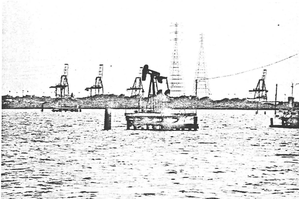
FIGURE 3-8. Submerged oil wells in the Goose Creek Oil Field near Baytown, Texas. These wells were once located on dry ground until subsidence in the oil field left them in their current, partially-submerged state.
