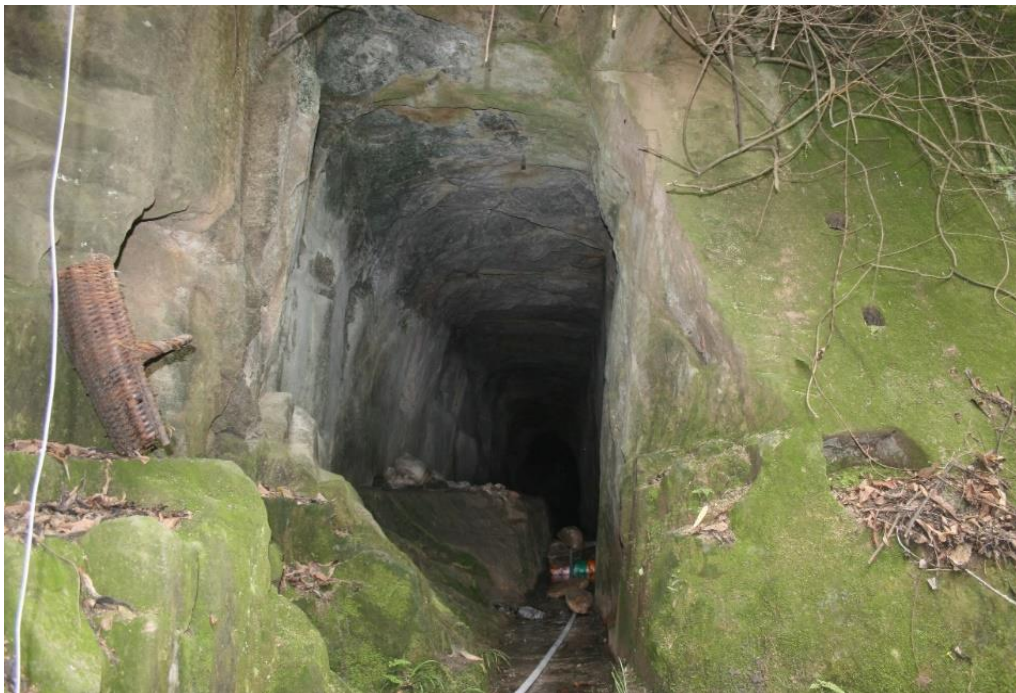
Fig. 60 Tunnel of coal mine at Liuhechang (photo by: Peng Wei)
