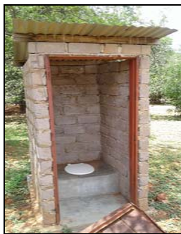
Fig. 6: A photograph image showing pit latrines. There is a pit latrine for each compound or household.
