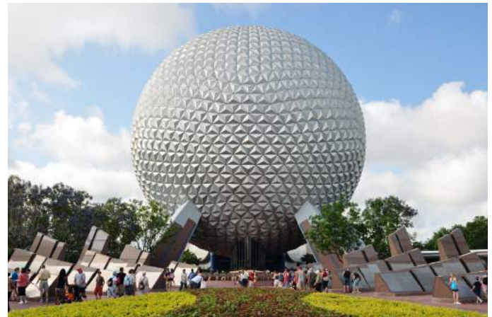
Fig. 24 Epcot Spaceship Earth Walt Disney World Orlando: Various triangles shape a strong structure in 3-dimension, By chensiyuan - chensiyuan
