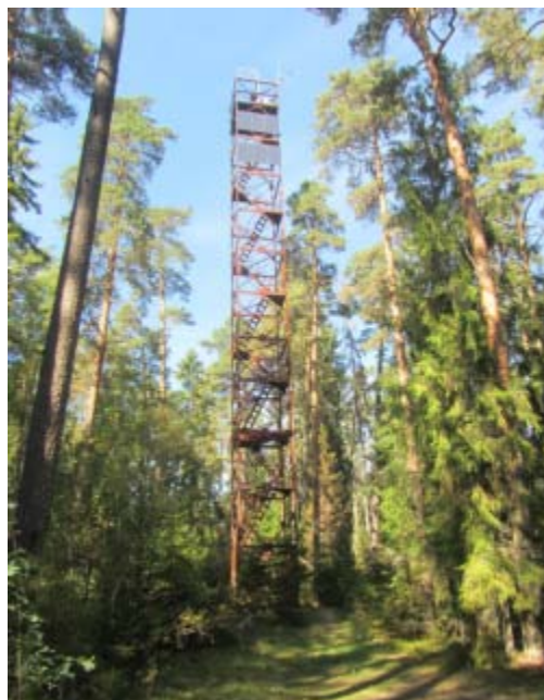
Photo 3. Observation tower for measurement on parameters
