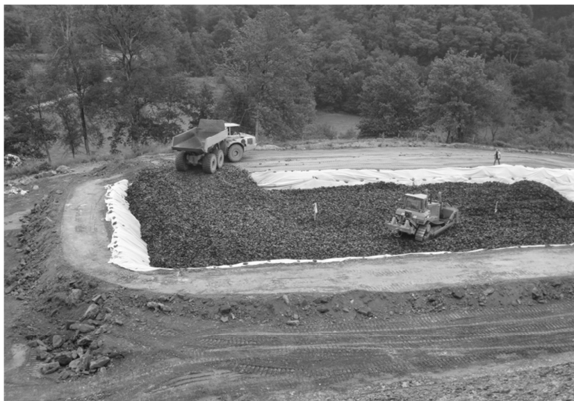
Figure 4. Construction of the TDA layer above the tunnel crown.
