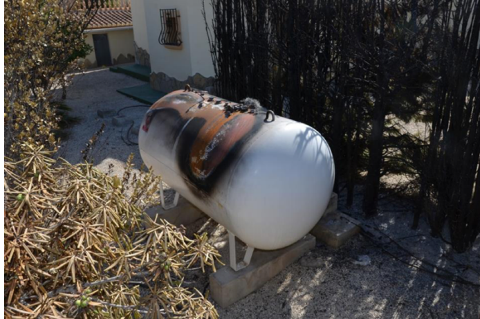
Figure 7. LPG damaged tank in Benitatxell fire (Valencia, 2016). Foto: David Caballero
