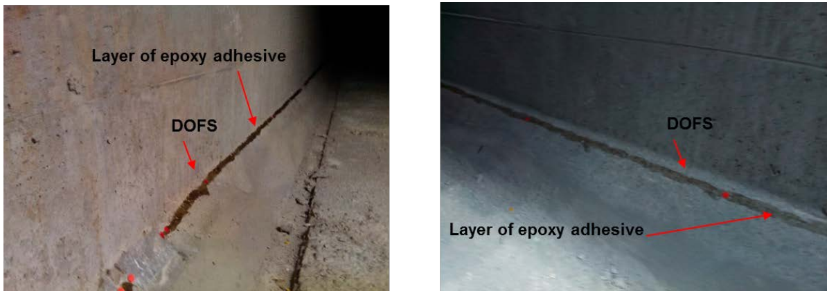
Figure 4. Final aspect of the sensor installation in Sarajevo Bridge
