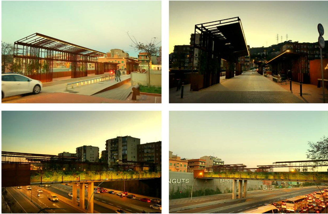
Figure 34. Sarajevo bridge after the completion of the rehabilitation works
