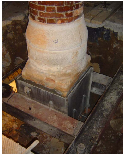
Figure 7. Preparation of columns to be replaced in this procedure
