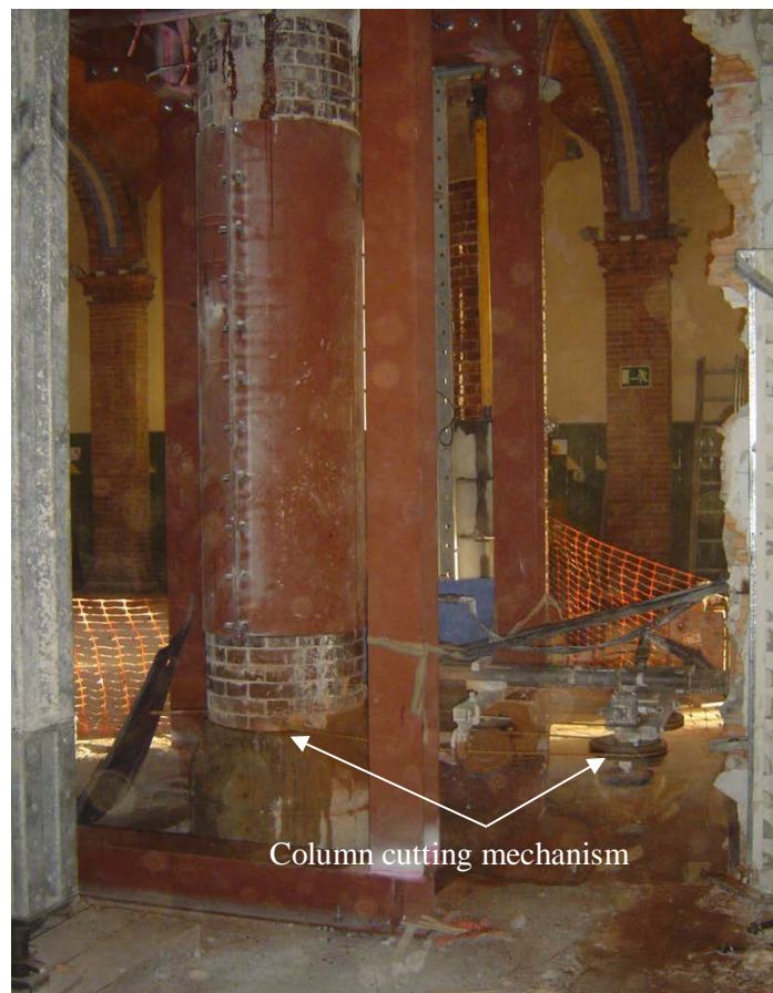
Figure 8. Cutting procedure of the columns
