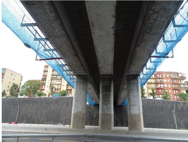
Figure 19. Bottom perspective of the bridge slab's box-girders
