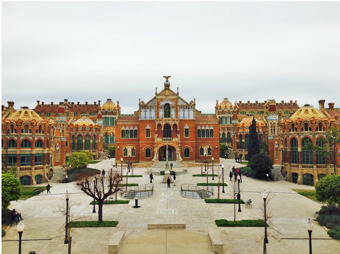
Figure 5. Sant Pau Hospital at Barcelona, Spain
