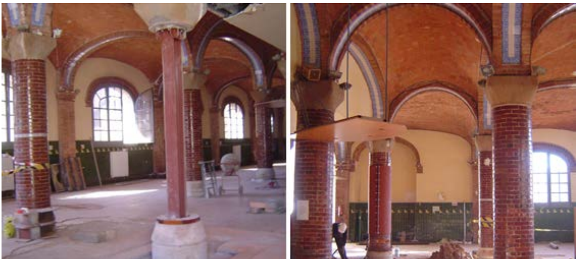
Figure 10. Final works. Implementation of steel profiles and following encapsulation
