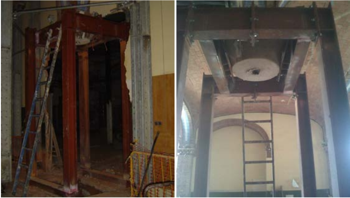
Figure 9. Temporary steel frame installed close to the columns to be replaced
