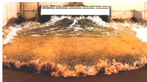
Figure 3. Flushing gate opening in a cleaning operation.
