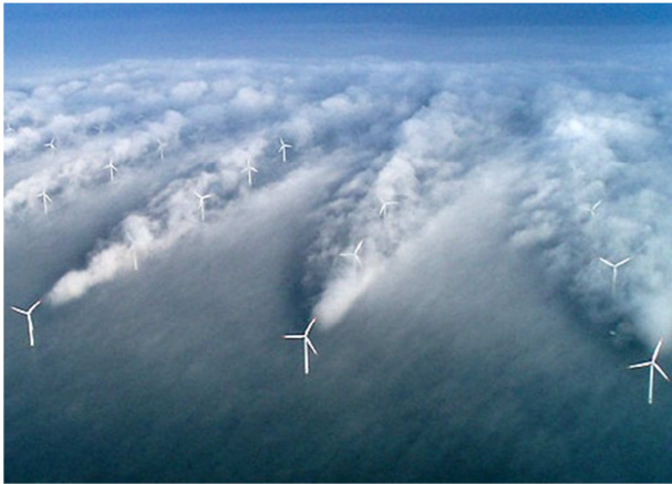
Figure 10: Array of wind mills in the ABL, with their wakes marked by condensation of water vapour
