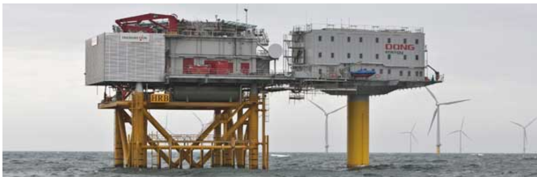
Figure 11. Poseidon (right), the first offshore wind farm accommodation platform in the world. Source: (Maritime Denmark, 2013)
