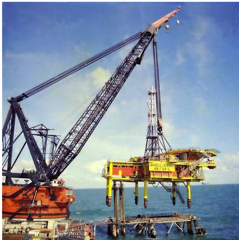
Figure 121. O&G platform being decommissioned in the North Sea. Source: https://www.oilandgaspeople.com/
