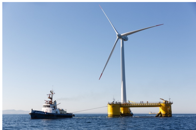
Figure 39. Wet tow of fully assembled and commissioned WF1 to installation site.
