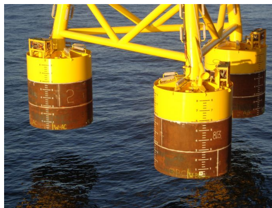
Figure 28. Jacket-structure equipped with suction buckets for Aberdeen Offshore Windfarm, Scotland. Source: http://www.indepthnrg.com/aberdeen-offshore-wind-farm/ /Figure 2 with suction.
