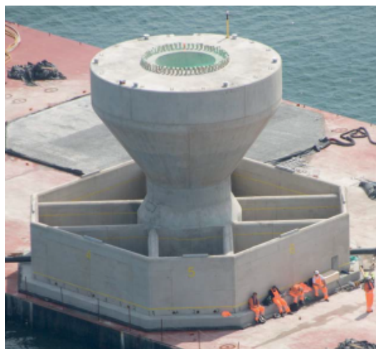
Figure 24. Gravity base foundation waiting to be installed.
