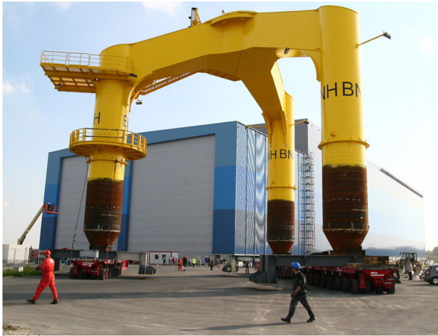
Figure 27. Tripile foundation for 5 MW Engineered by Bard
