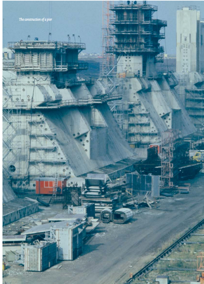
Figure 57. Pier in construction dock.
